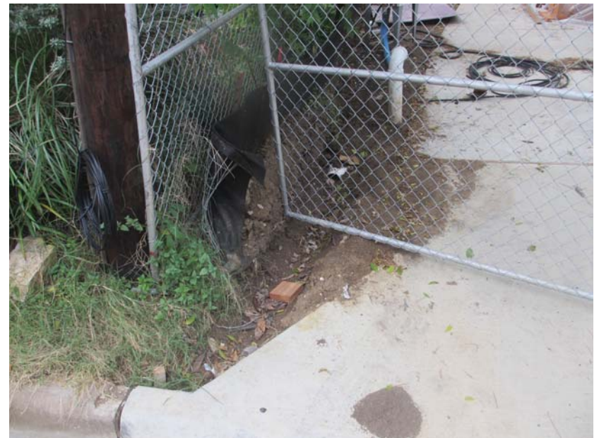
1819 Treadwell - no controls at the lowest corner on the lot allows sediment to escape; erosion channel readily visible
