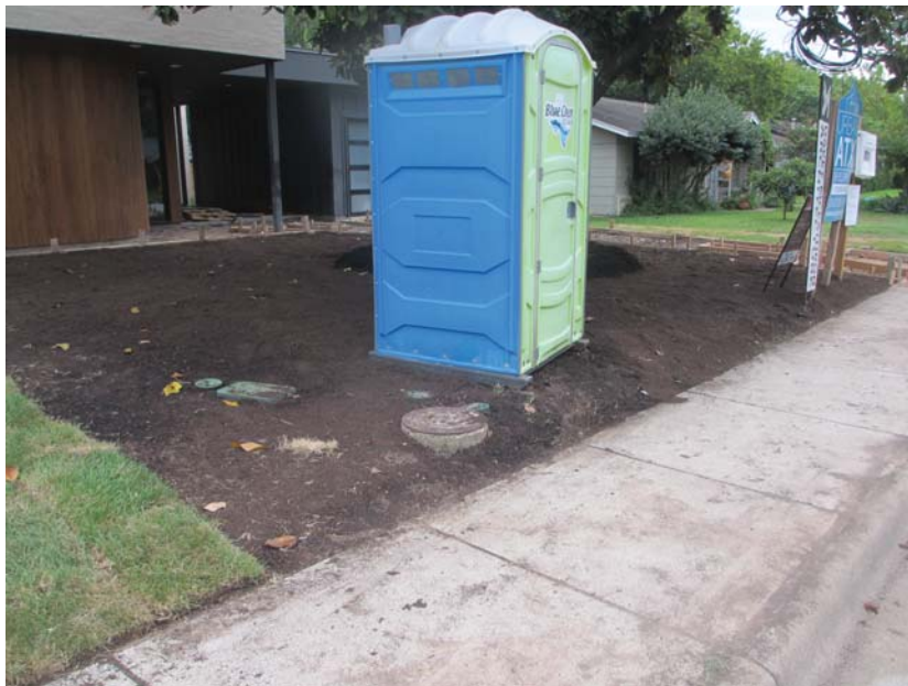
1811 Ashby - no controls; LDC § 25-8-181 requires controls to remain in place until permanent revegetation has been established
