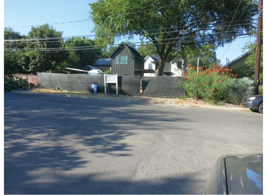
1610 Hether - Lack of erosion controls is hidden by the privacy fence.
