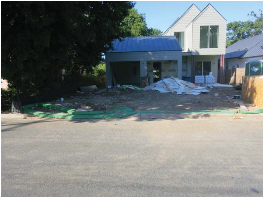
2012 Rundell (BSZ) - Flattened mulch sock will not prevent sediment from escaping.
