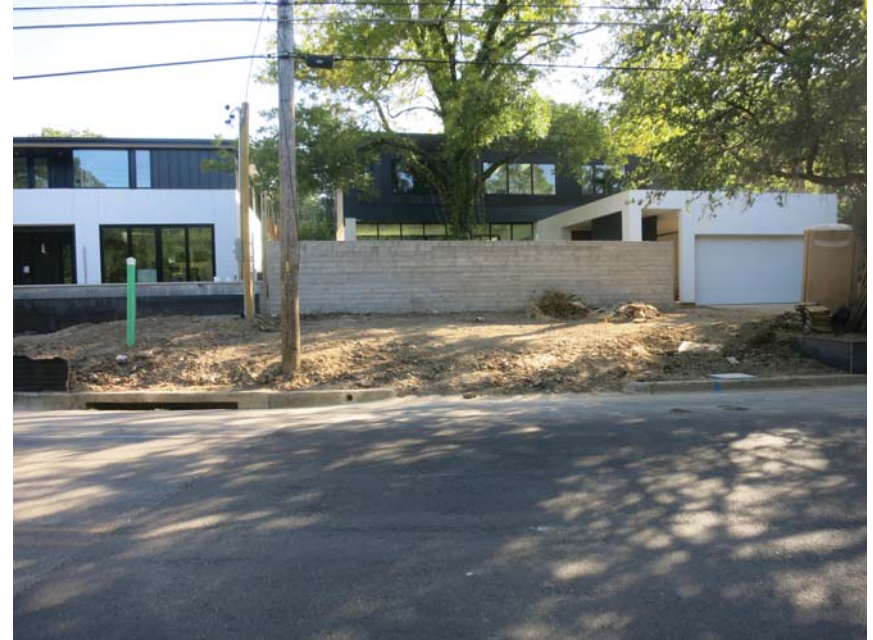
2005 Melridge (BSZ) - No controls. Multiple repeat offender. Storm sewer discharges directly to Little Zilker Creek.
