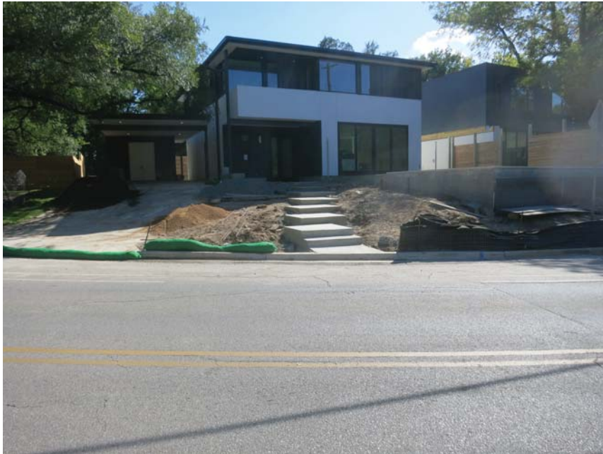
2003 Melridge (BSZ) - The controls do not extend along the entire frontage. Multiple repeat offender a few feet from Little Zilker Creek.
