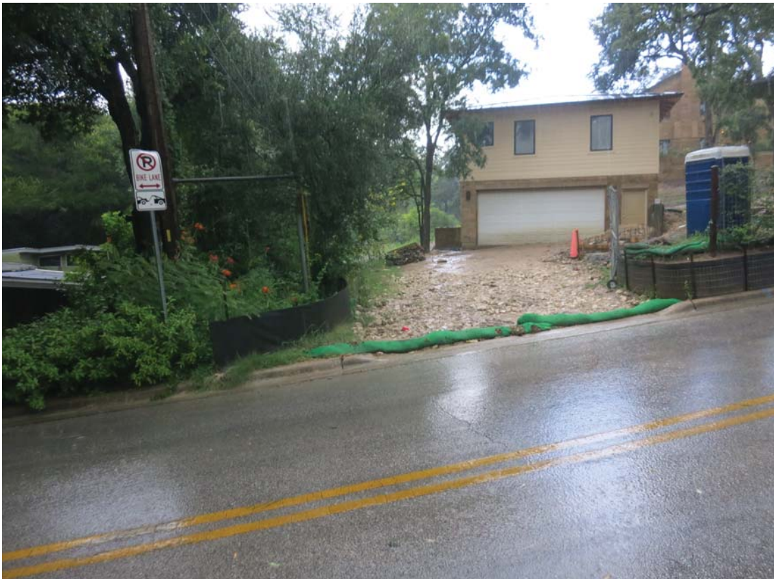
1113 Azie Morton (in the Barton Springs Zone) - Insufficient controls on steep slope.
