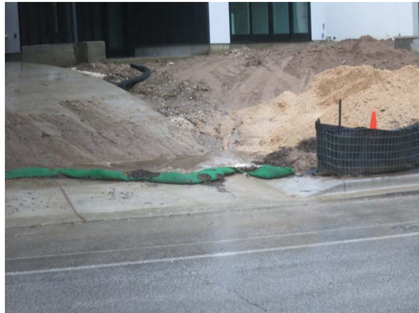
No j-hook in silt fence to extend up driveway. Insufficient controls on steep slope. Sediment has overtopped mulch sock.
