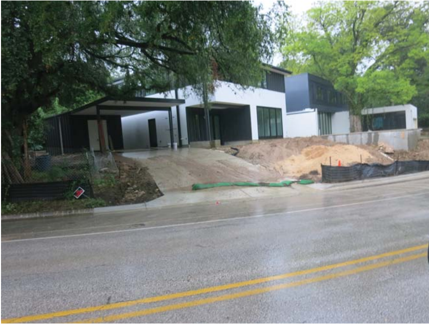
No j-hook in silt fence to extend up driveway. Insufficient controls on steep slope. Sediment has overtopped mulch sock.
