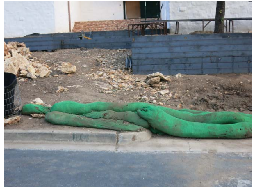
Mulch socks stacked on top of each other (prohibited by specs). No staking of mulch socks. No j-hooks. Slope too steep for one row of mulch socks.
