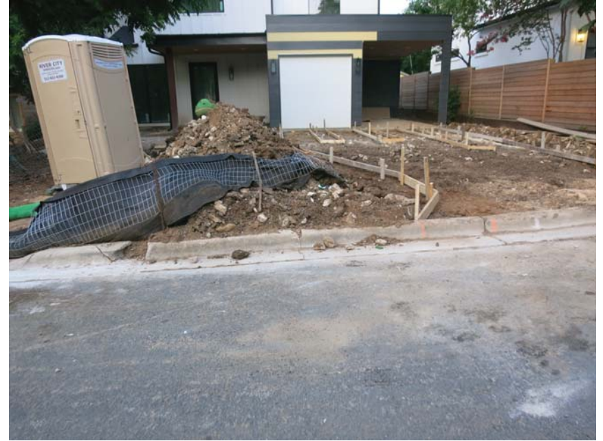
2109 Peach Tree - No controls for dirt between mangled silt fence and curb.
