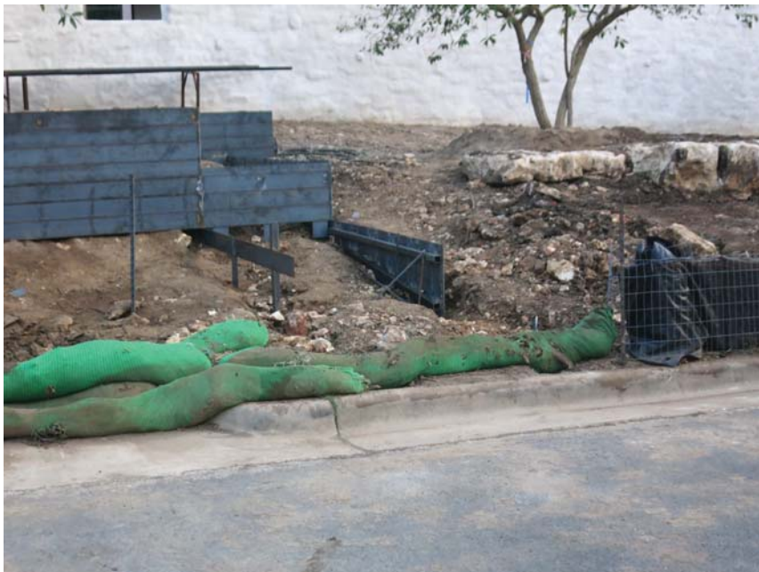
Mulch socks stacked on top of each other (prohibited by specs). No staking of mulch socks. No j-hooks on mulch socks or silt fence. Slope too steep for one row of mulch socks.
