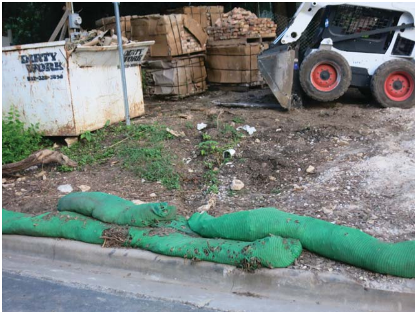
Mulch socks stacked on top of each other (prohibited by specs). No staking of mulch socks.
