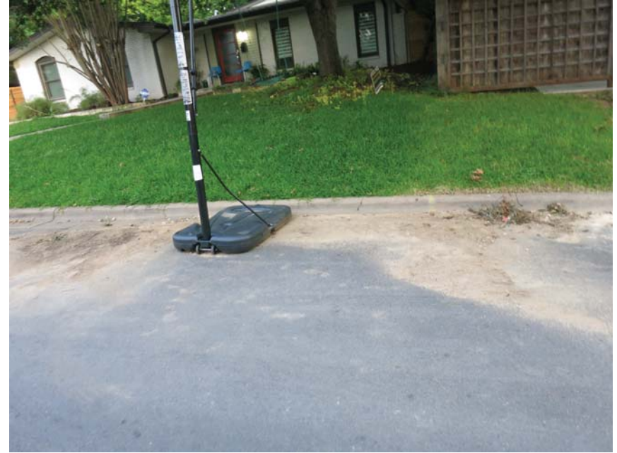
2112 Ann Arbor - Sediment deposited in street downstream of 2112 Ann Arbor.
