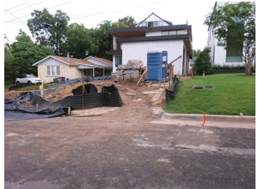
2019 Ashby - however, on right side of site there are no controls; there is a direct path to gutter and street for dirt and sediment to leave the property from this steep slope
