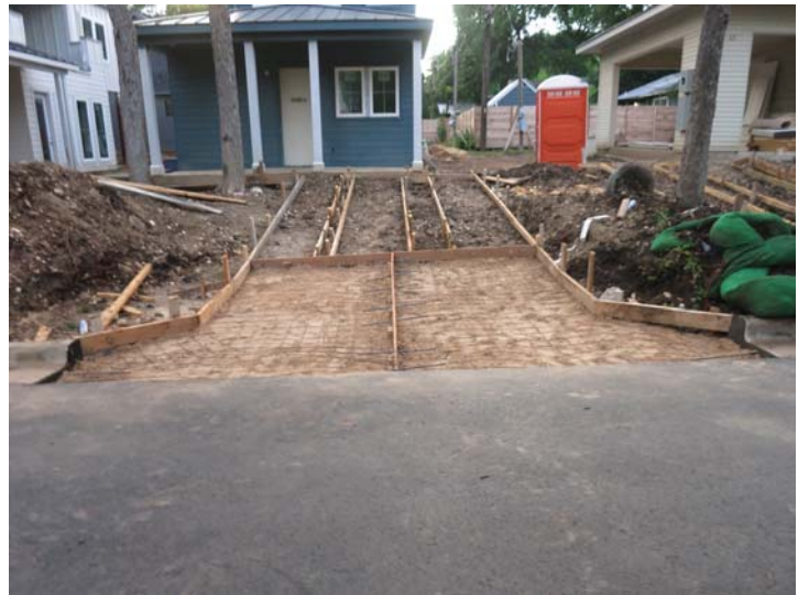
along Paramount - no controls for sand in driveway; if it rains sand, sand will erode
