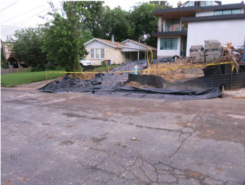
2019 Ashby - plastic sheeting has been properly placed over driveway forms and sand to prevent erosion
