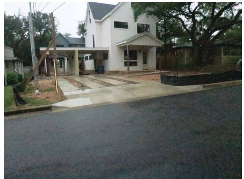
2207 Rundell - controls do not exist to prevent runoff and sediment from leaving site on left side and from ribbon strips
