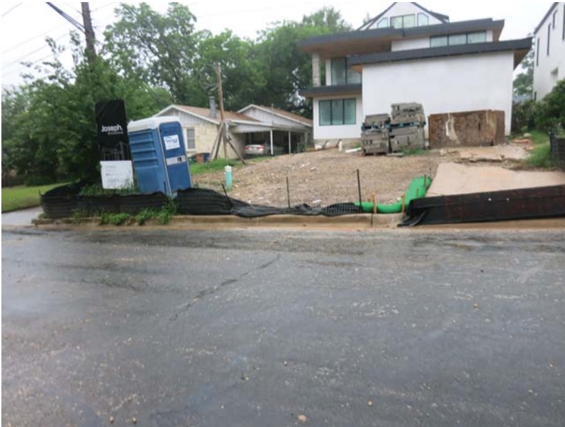
2019 Ashby - crushed silt fence
