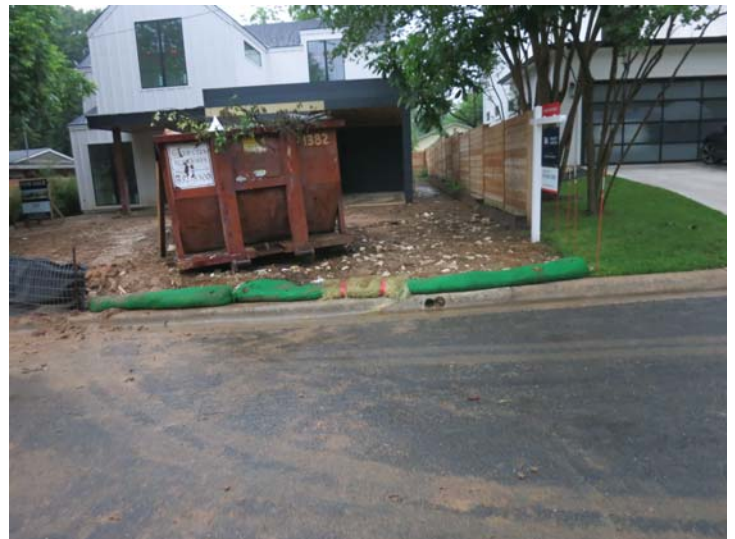
straw waddle unacceptable; hopefully just filling the gap until it is replaced
